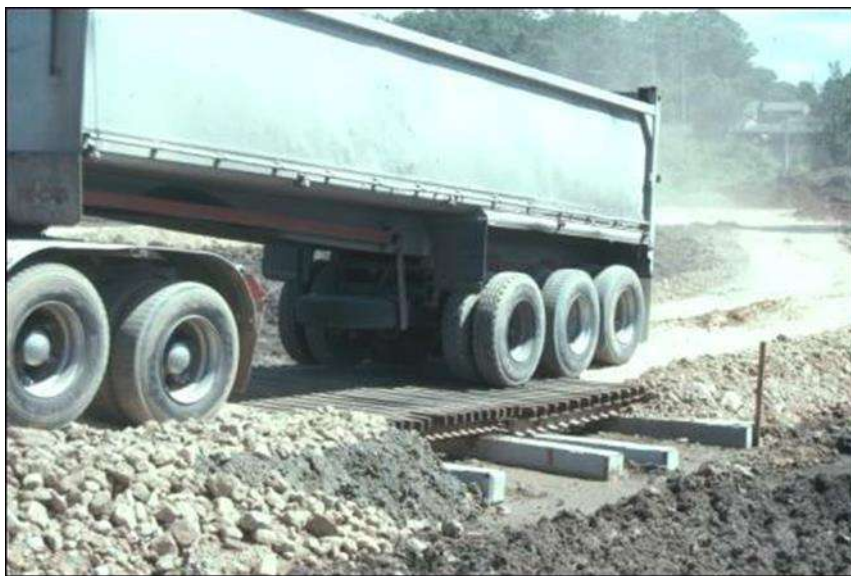
Figure 11 Rumble strip similar to that illustrated above will be placed at the main site access.
