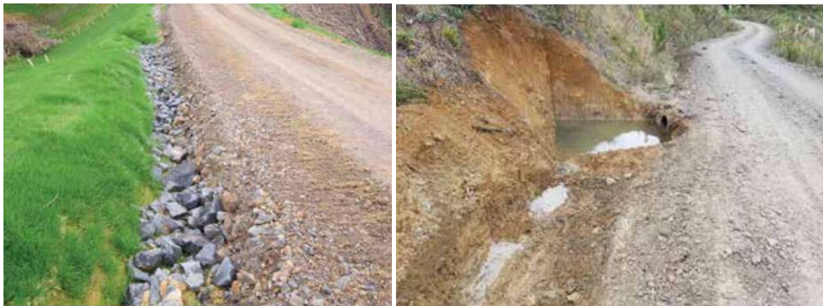
Figure 15 Example of energy dissipation rip rap (left) that will be employed in steep grade areas within the channel; and a sediment trap (right) that may be dug upstream of culverts. (Source: NZ Forest Road Engineering Manual).
