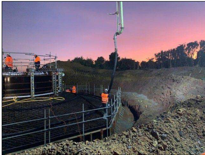
Figure 15 Example of a Tower Foundation Concrete Pour
