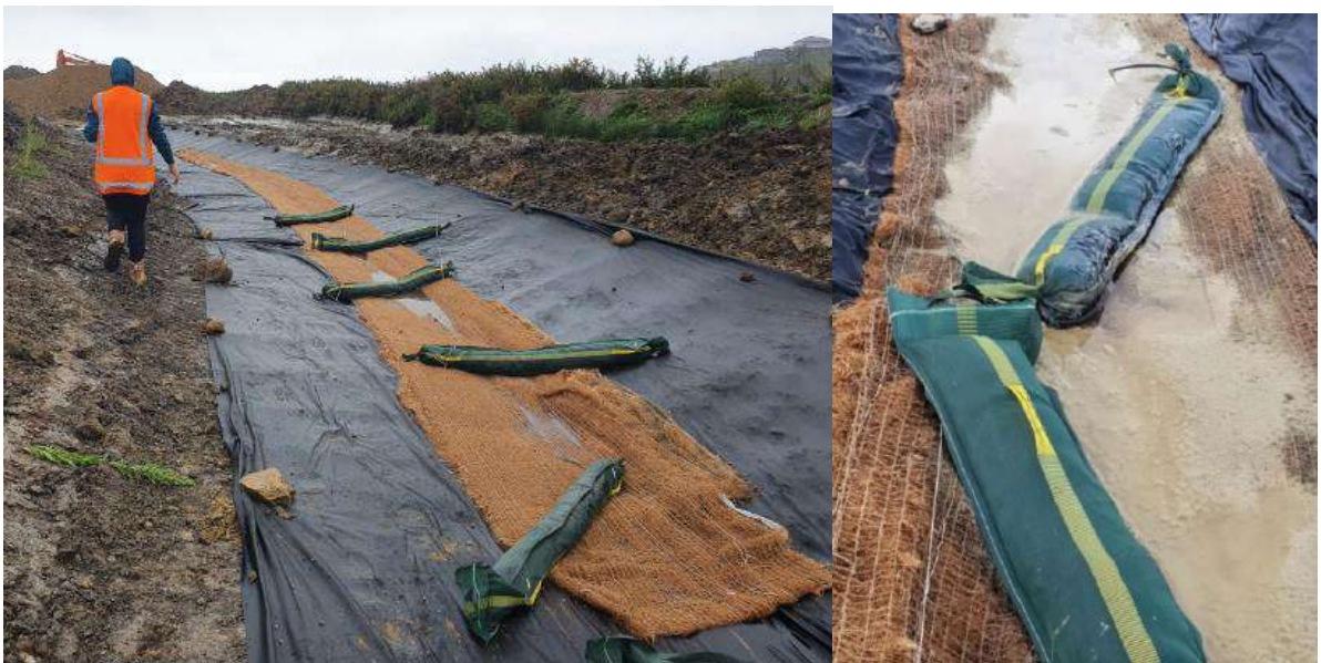
Figure 13 illustration of K-log channels and natural fibre matting successfully retaining fine sediment. (Source: EnviroCo)
