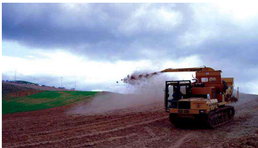
Figure 10 Straw Mulching to be Used in Conjunction with Surface Roughening.
