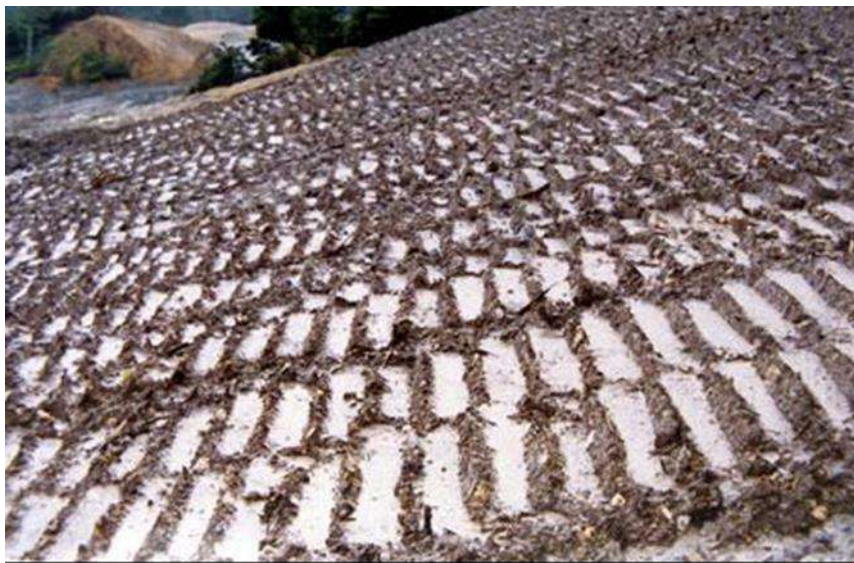
Figure 9 Soil Surface Roughening to be Employed Downstream of Areas Where the Soil has been Disturbed.
