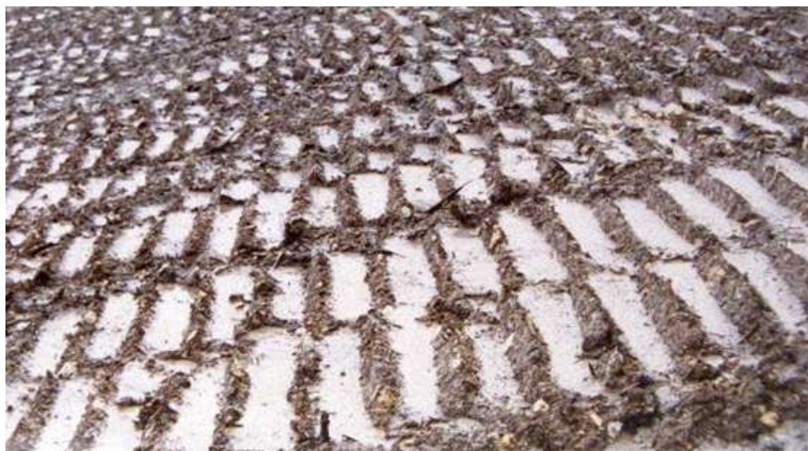
Surface roughening of a slope. Note that the hollows act as 'micro' sediment traps
