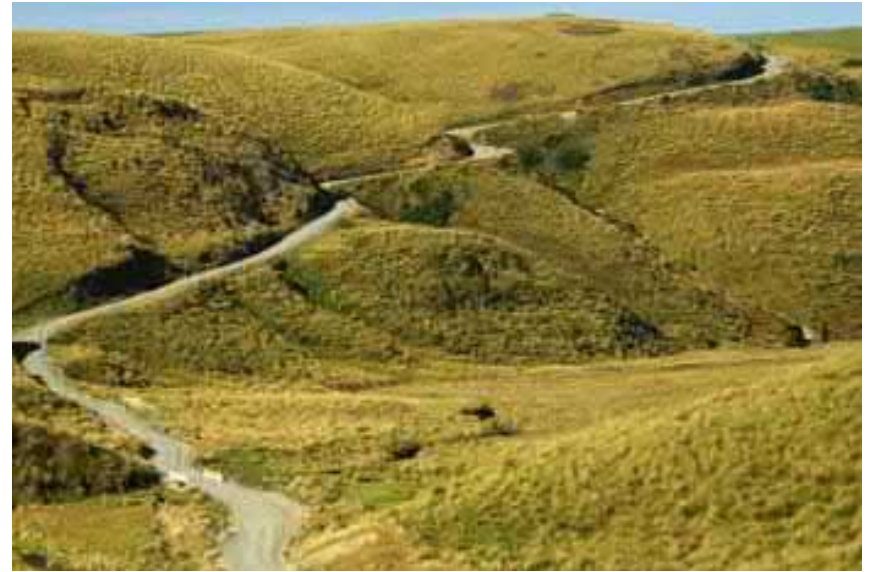
Fig. 46 An example of high-impact cuts and poor mitigation.
